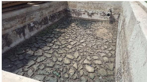
Plate 2. Almost dewatered FS (DFS) on the drying bed
