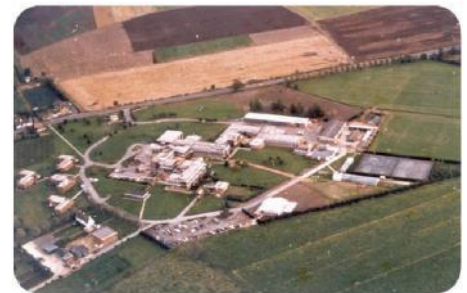
National College of Agricultural Engineering at Silsoe
