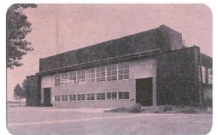
Hanger conversion into laboratories
